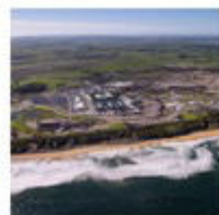
Victorian Desalination Plant Warragul, Victoria, Australia
