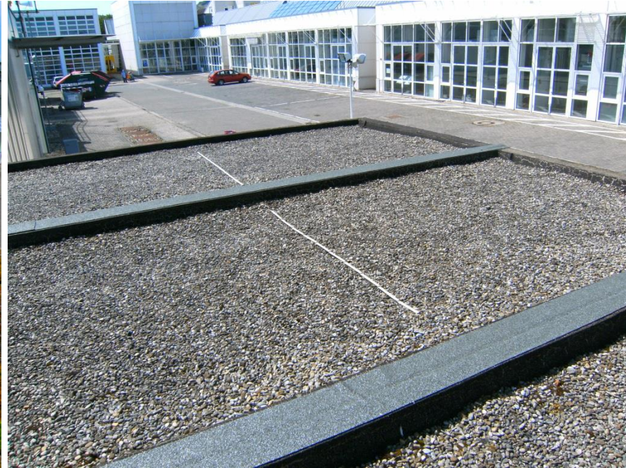
Bitumen and 3 - 5 cm gravel
