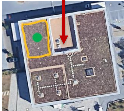
Cool roof, Mainz
