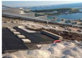
Protectodrain® and Elastodrain® mats ensure the safe drainage of exceeding water on the entire surface.
