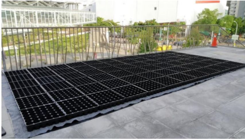
Lay the drainage board
