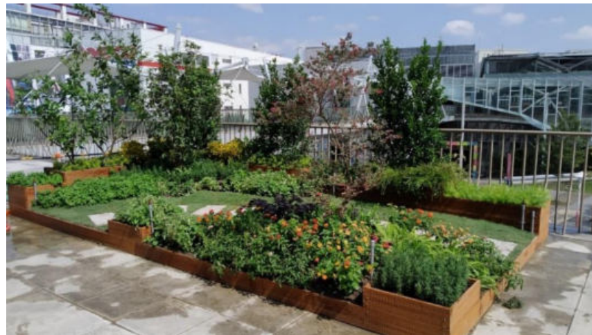
installation of carbonized bamboo boards/ Plants
