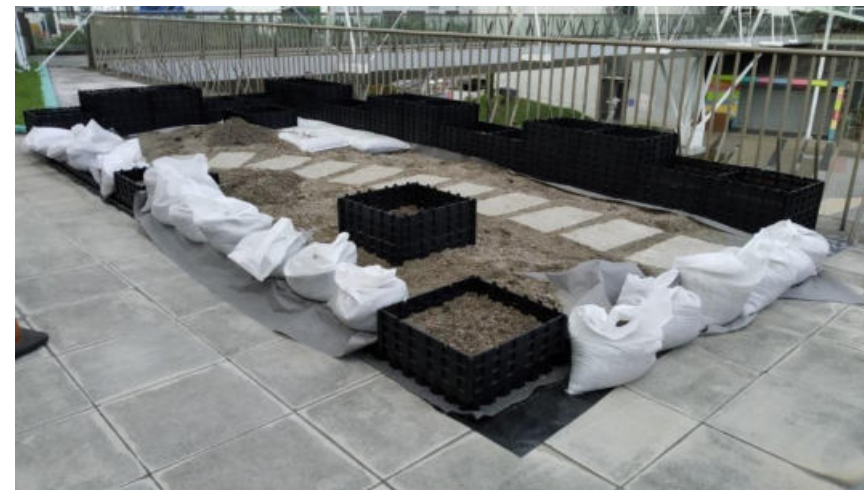
Lay filter blanket and lightweight soil
