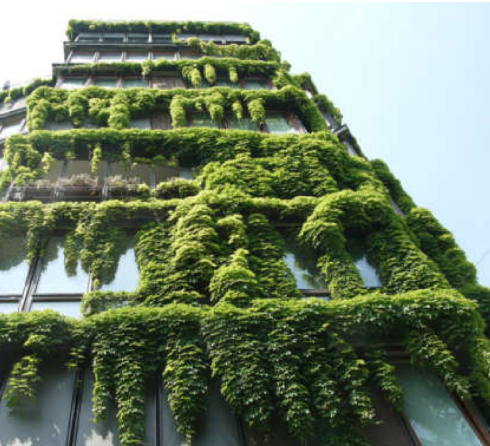
unknown project in Milan
